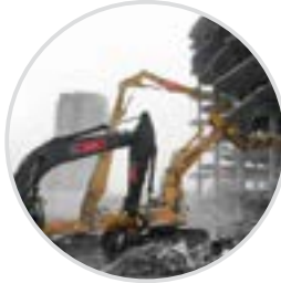
DEMOLITION & SITE CLEAN-UPS ↗
